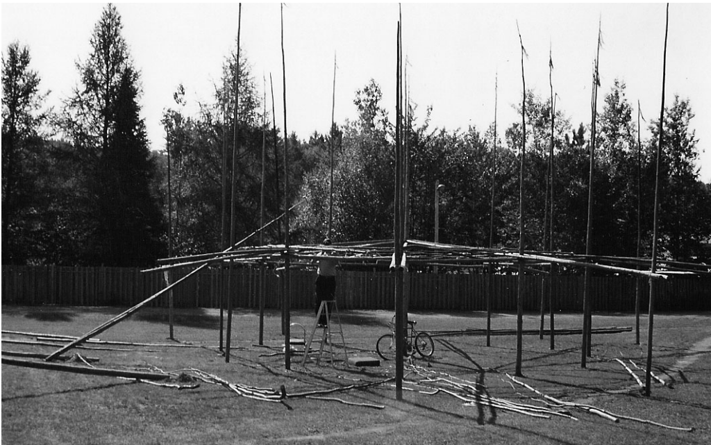
Building the arbor for community circles.
